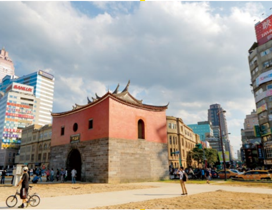
The Beimen Access Road Removal is the first step in the “West District Gateway Project.” (Photo: Daniel M Shih)
