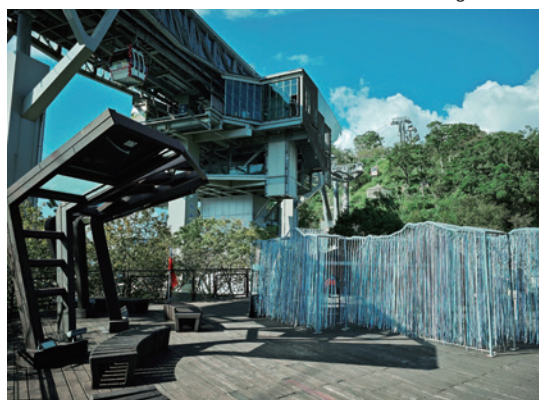
Green Ray Platform beside gondola station
